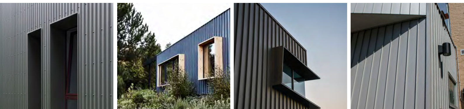
Figure 23: Sheet piling as side cladding examples.
