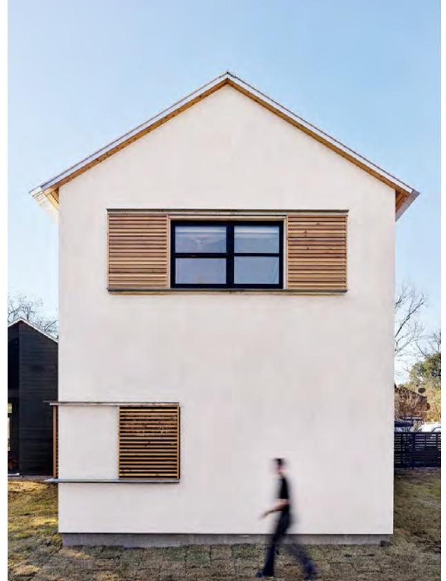
Figure 43: Timber sliding shutters
