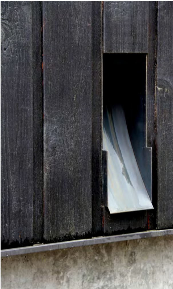
Figure 29: Hiding gutters and downpipes
