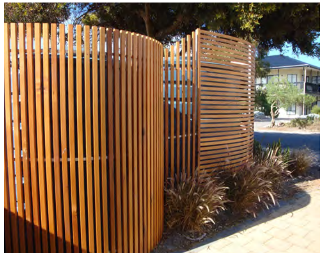
Figure 46: Timber slats used to conceal rainwater harvesting tanks
