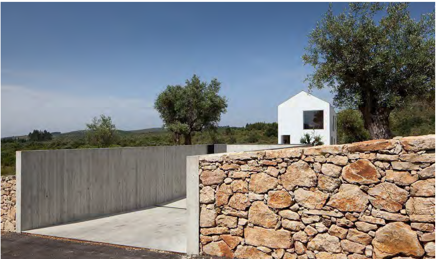
Figure 19: Retain structure materials collage
