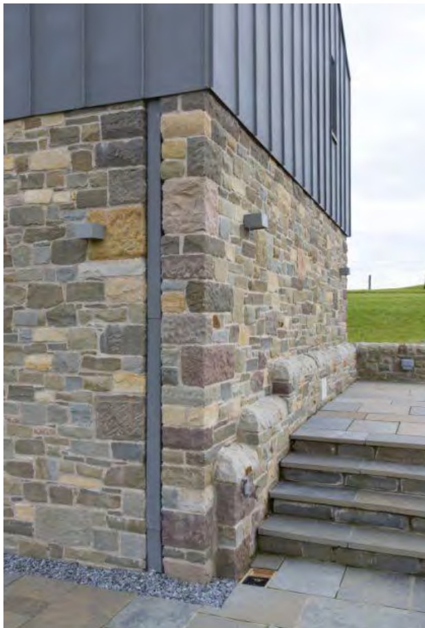
Figure 28: Hiding gutters and downpipes
