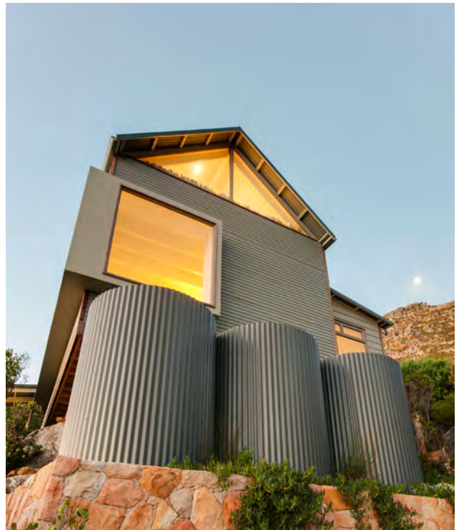
Figure 47: Corrugated sheets used to conceal rainwater harvesting tanks
